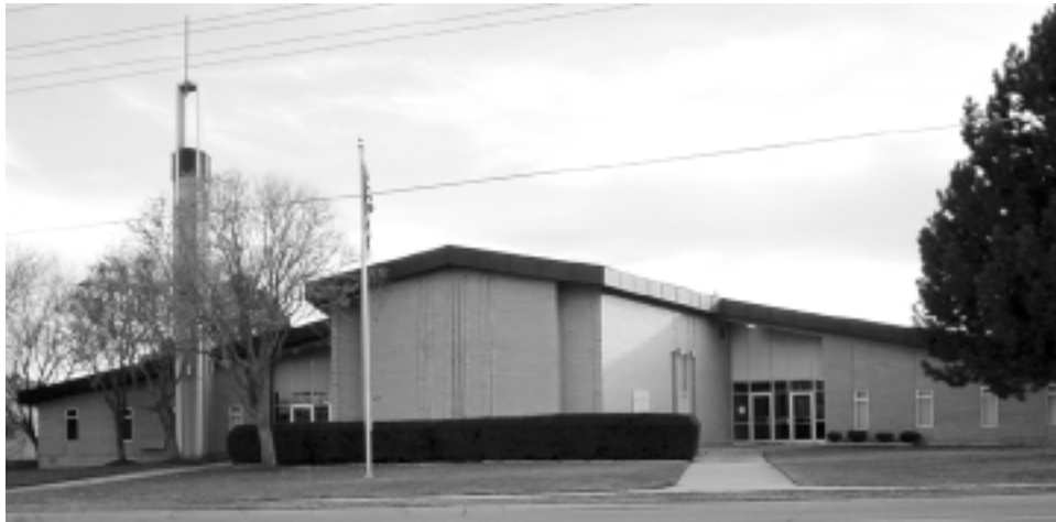
The Current West Jordan 4th Ward and Stake Chapel 1899 West 7600 South, West Jordan, Utah
